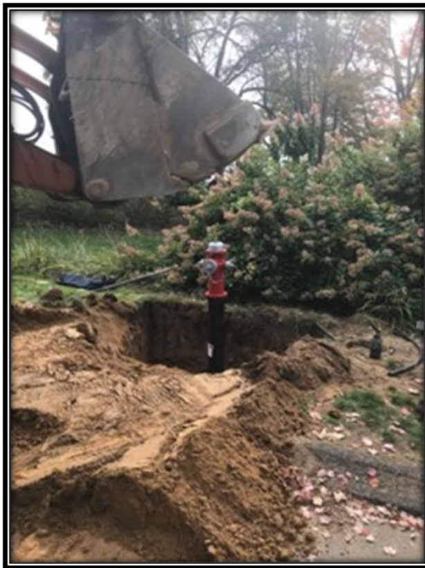
New Hydrant - Chapel Hill
