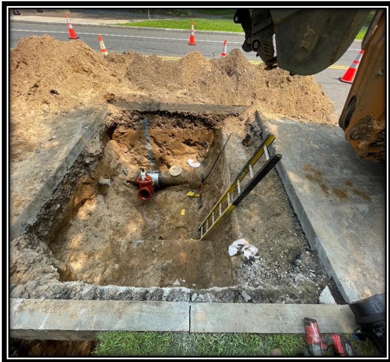
Tie-in for Service to Pearson's Hall Mount Holyoke College
