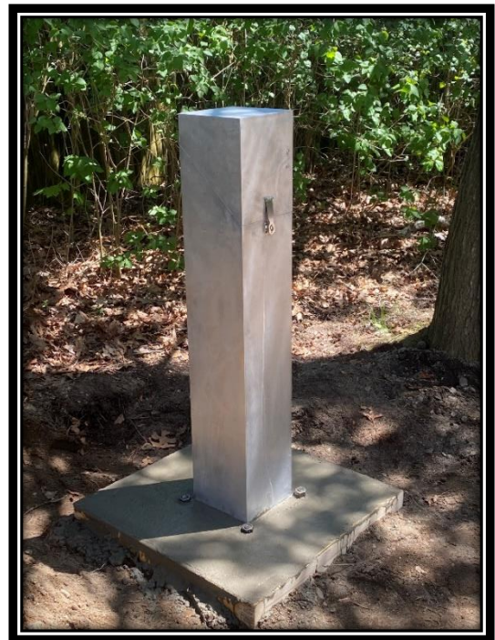
Sampling Station Woodside Terrace
