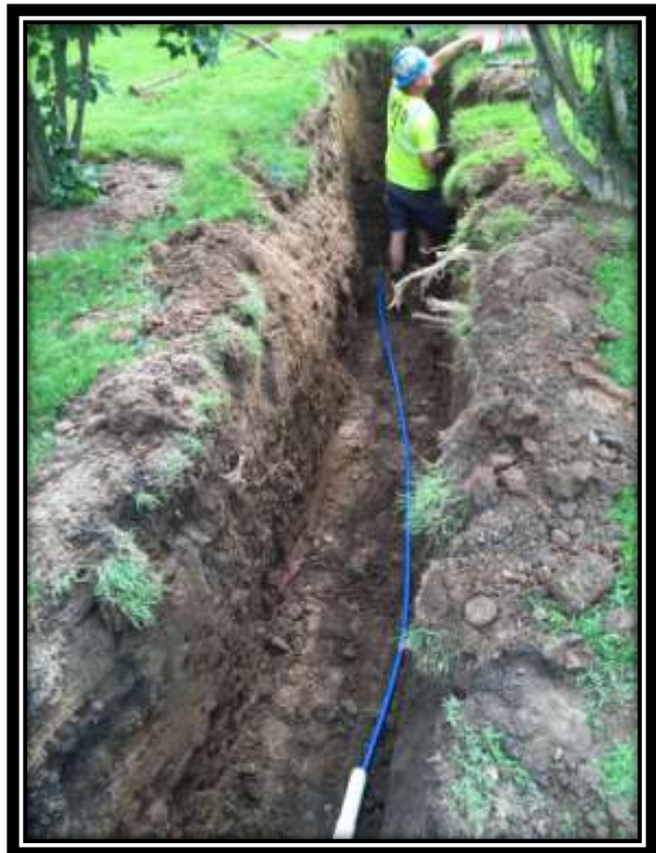
Todd Calkins, Water Systems Operator, Installing a Water Service Line on East Street
