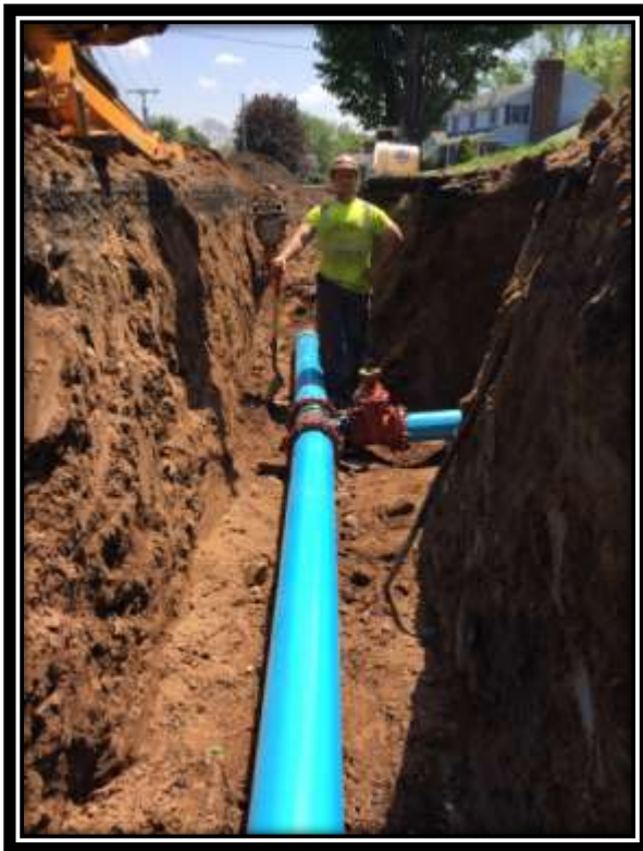
Tyler Scheinost, Water Systems Operator, Installing a Hydrant on East Street
