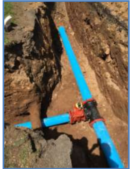
Installing Hydrant Tee
