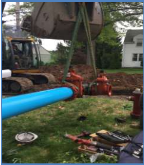
Installing Hydrant Tee
